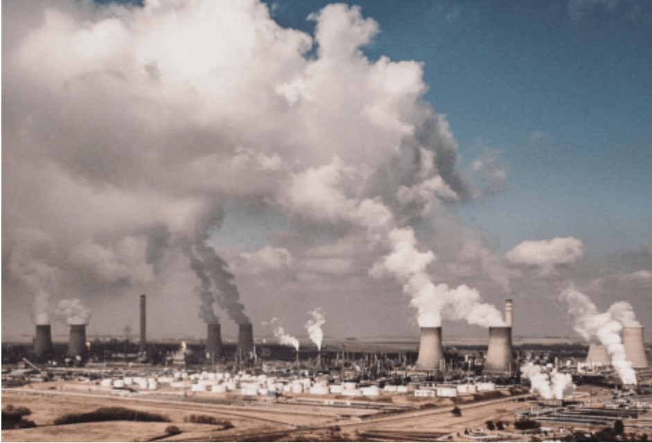
Sasol's Secunda mega-plant (Photo by Alexander Glustrom)
